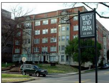
The Blackstone apartment building with its 48 units dates to the late 1920s and is now one of the most visible older structures identifying West End Park. The neighborhood signs were purchased with a city grant received by the West End Park Neighborhood Association in 2003. (GEORGE ZEPP / FOR THE TENNESSEAN)
